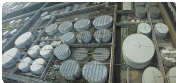
Wastewater treatment plant (After improvement)
